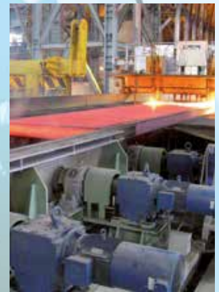
NORD drive units in a steelworks.
