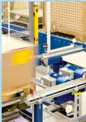
NORD drives in the high rack storage area in Bargteheide.
