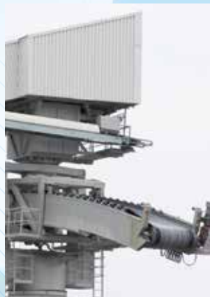
NORD drive units in the NorStone AS gravel plant in Norway.
