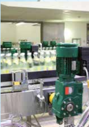
NORD drive units used in a bottling plant in a South German brewery.
