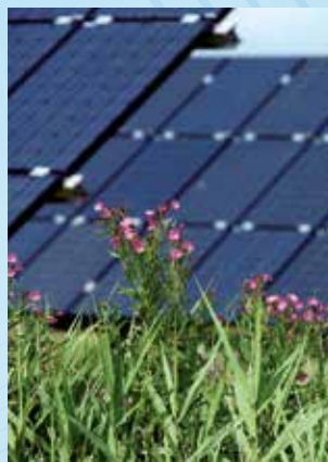
At the Rodenäs Solar Park, NORD drive units move the solar panels to track the sun.
