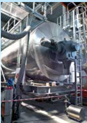
NORD drives in use at Dong Energy, a Danish energy supplier.
