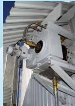
NORD drive units in a biogas plant.
