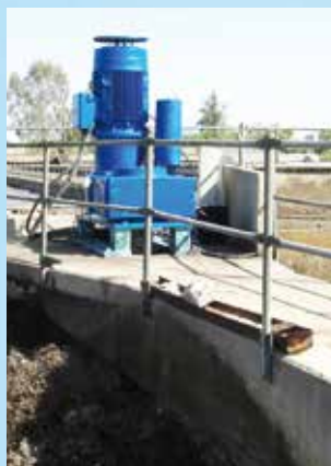
NORD drives in a sewage treatment plant in Tunis.
